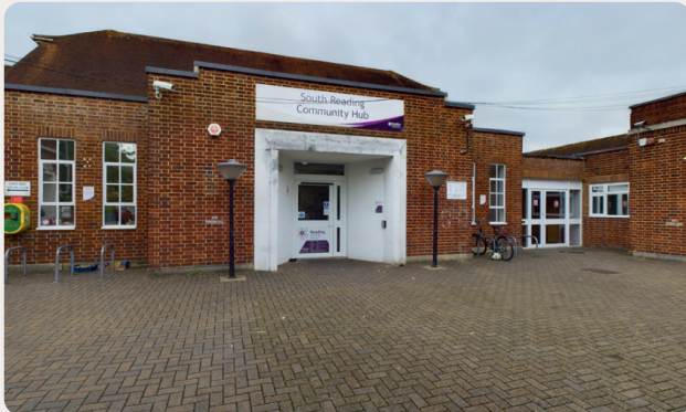
South Reading Family Hub 252 Northumberland Ave, Reading RG2 7QA
